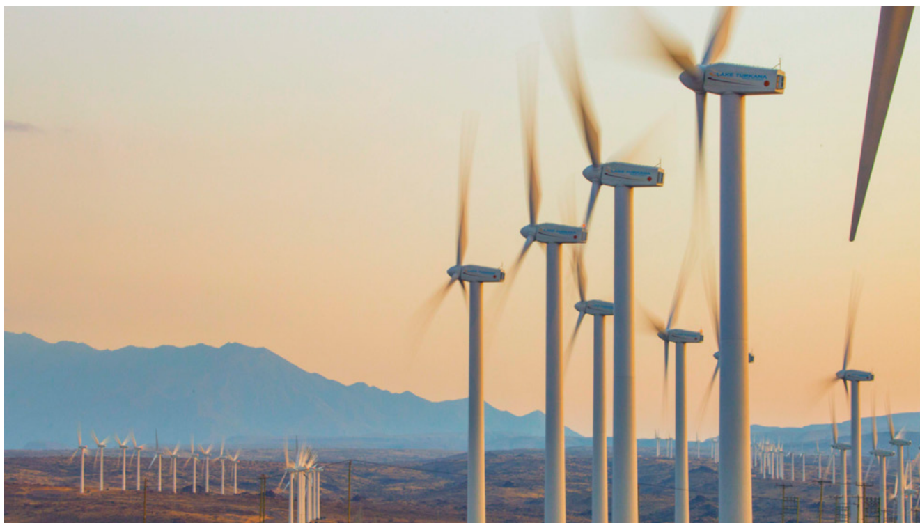
In 2018, Africa's largest wind farm Lake Turkana Wind Power was connected to the national grid. Finnfund has been a shareholder in the company ever since the construction began in 2013.
