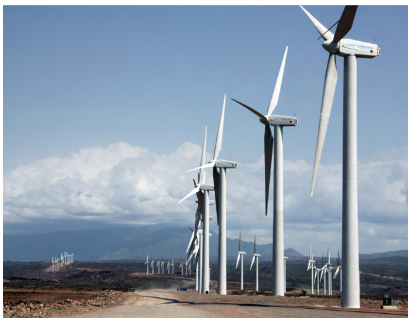
Lake Turkana Wind Power, with a total capacity of 310 megawatts, is the largest wind park on the African continent and the biggest single private sector investment in Kenya's history. Finnfund invested in Lake Turkana Wind Power in 2013. Photo: LTWP
